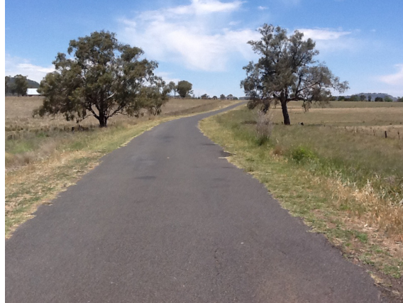
Photo of Gaspard Road looking North. Site on Left.
