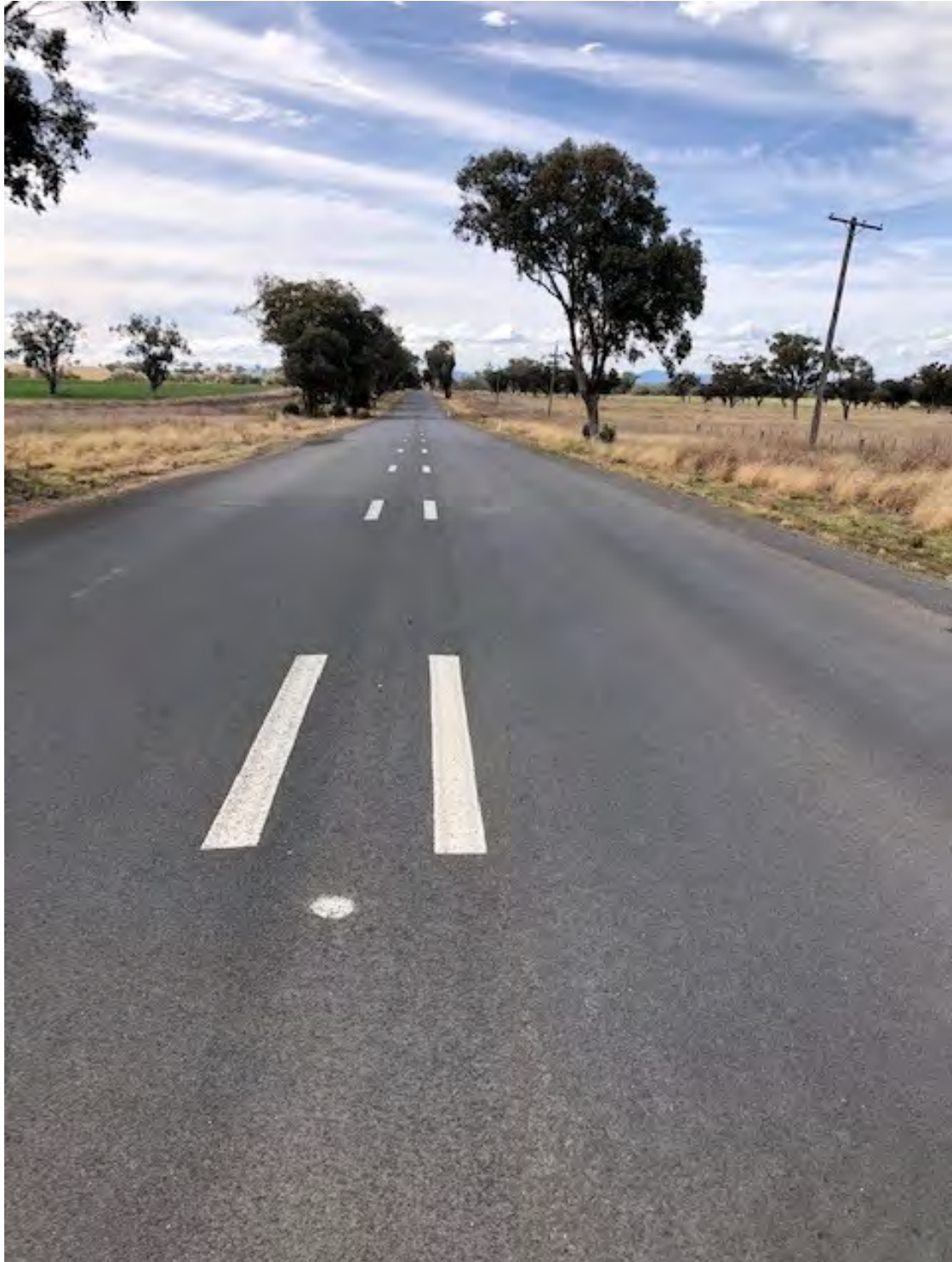
Plate 7 – New style of line-marking on Werris Creek Road with widened centreline marking
