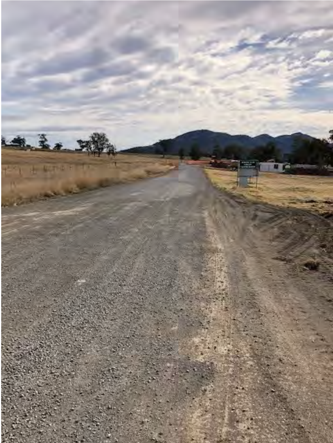
Plate 3 – Currabubula quarry access road viewed towards the intersection with Werris Creek Road
