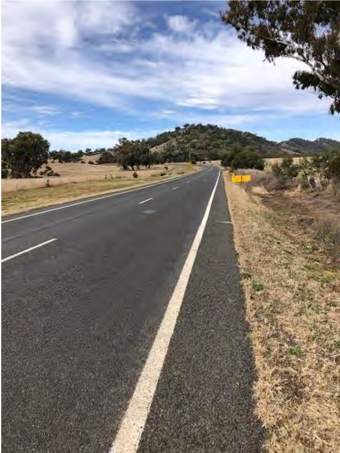
Plate 6 – Typical alignment of Werris Creek Road
