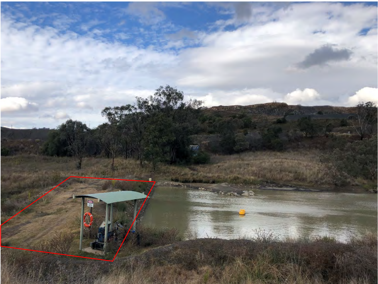
Figure 10 – Existing sediment basin embankment
