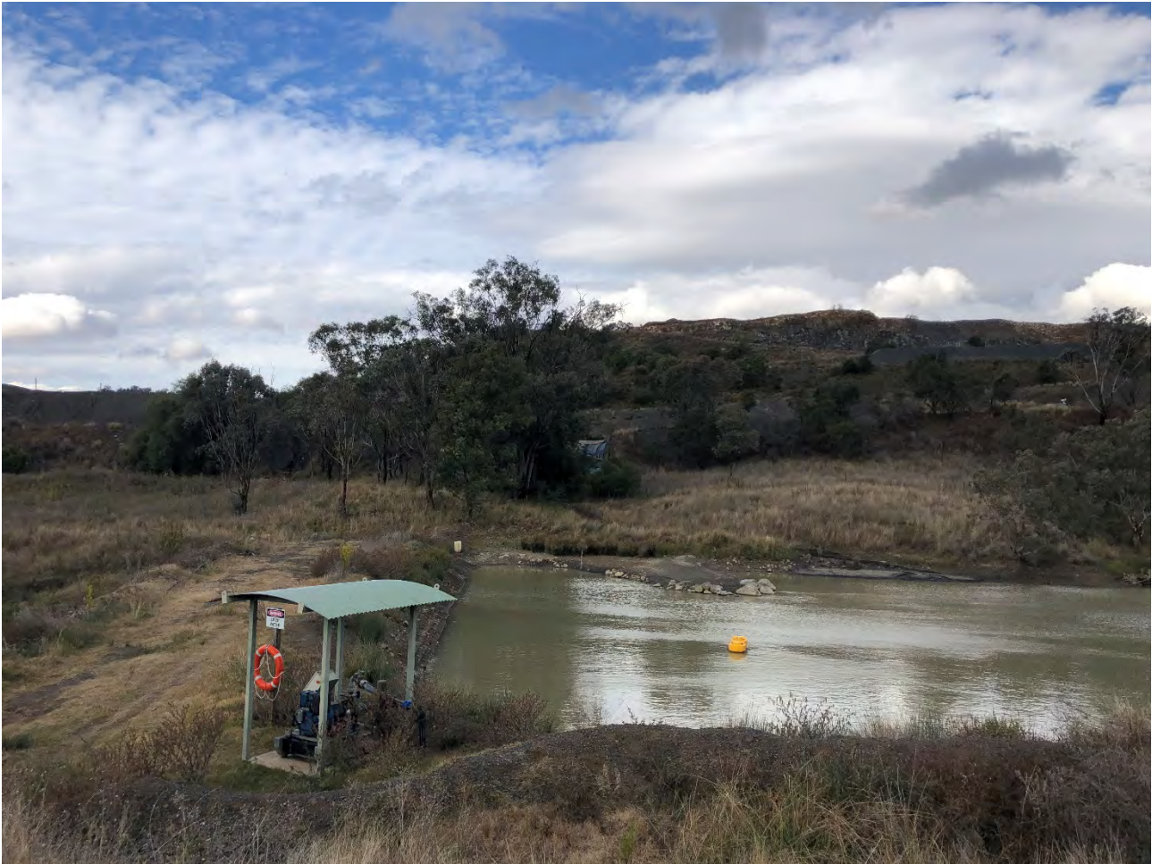
Figure 9 – Existing sediment basin and embankment
