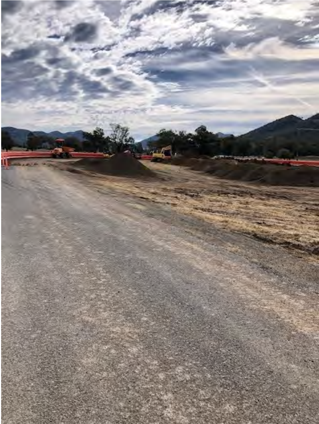
Plate 4 – Intersection works for the quarry access road on Werris Creek Road
