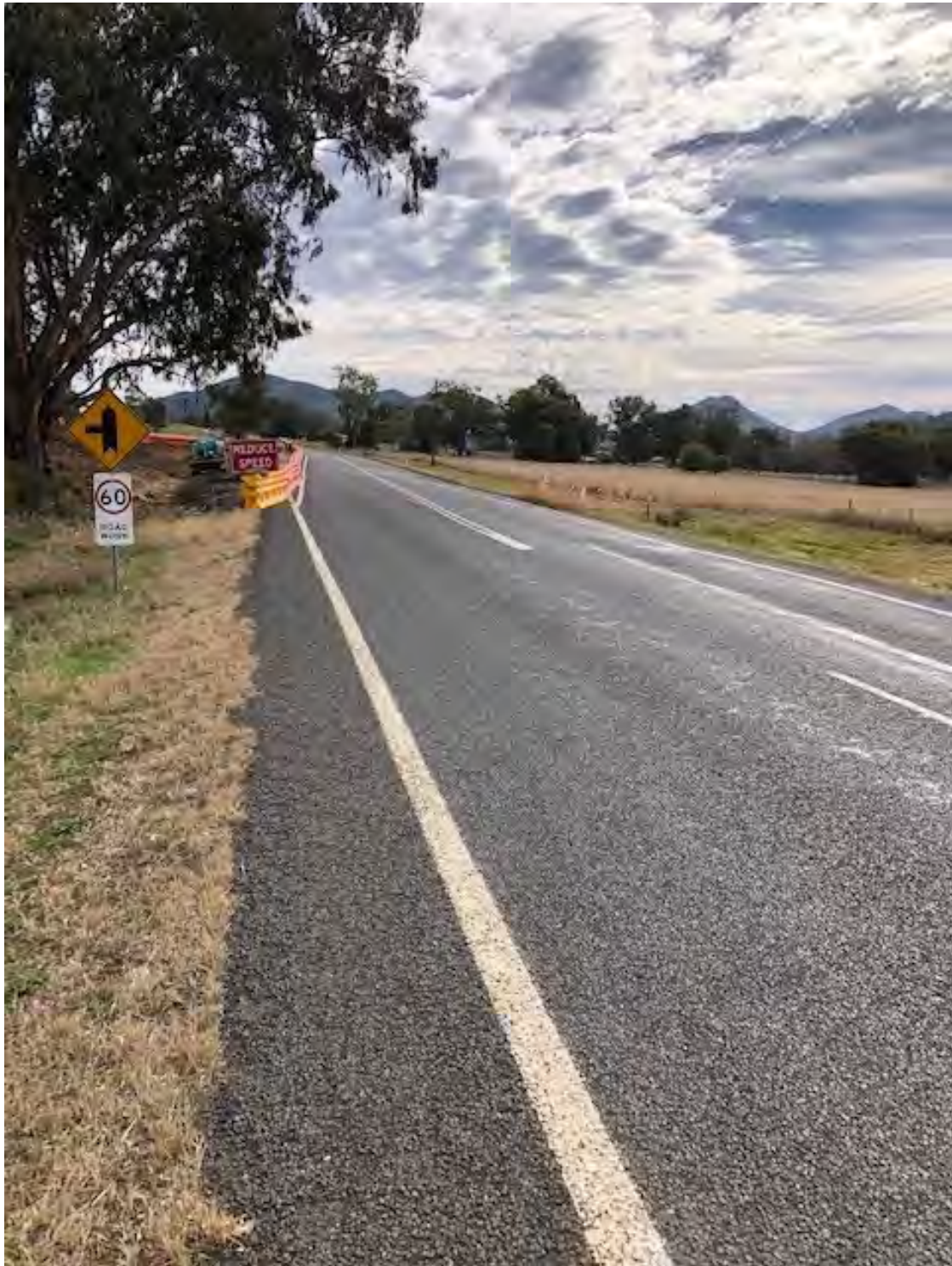
Plate 5 – Intersection works for the quarry access road on Werris Creek Road
