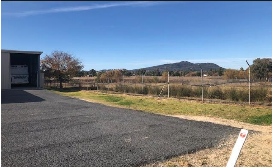
Figure 2: View of the Shed facing South-East (Source: Howards Bus Pty Ltd, 2023)
