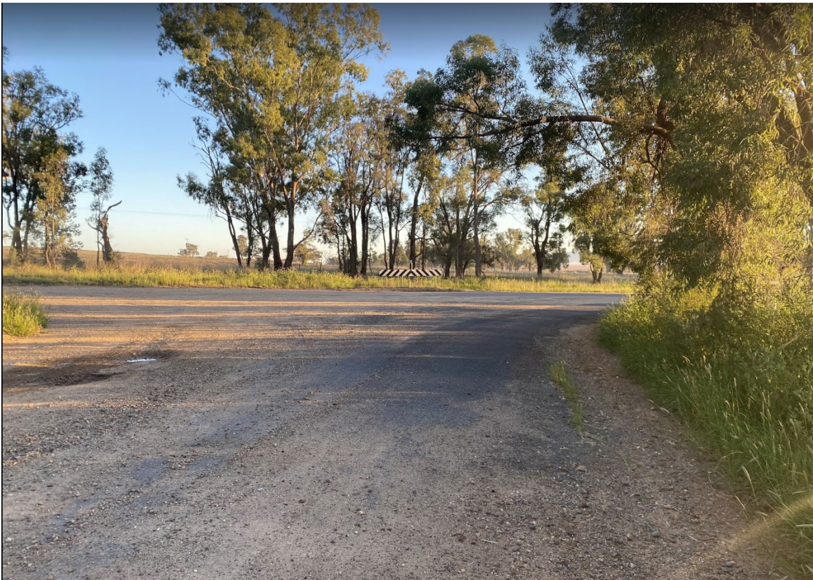
Figure 7: Inverkip Road looking North (Source PSA Consulting, 2022)
