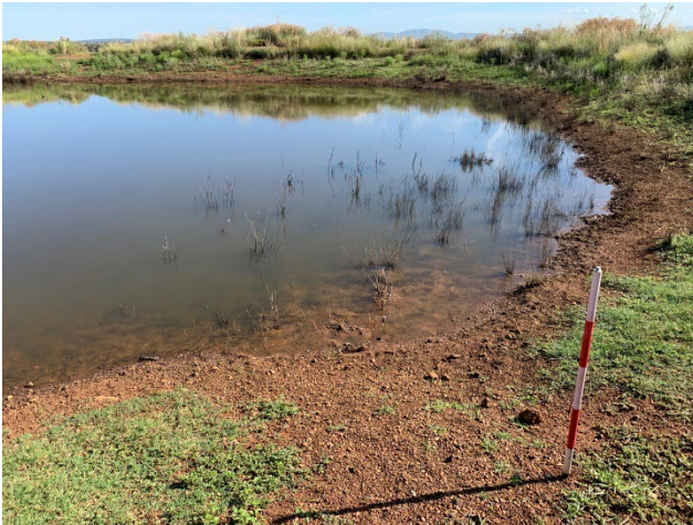
Plate 12: Dam central to Activity Area with an old windmill. Table drains surrounding the dam for water direction, facing east.
