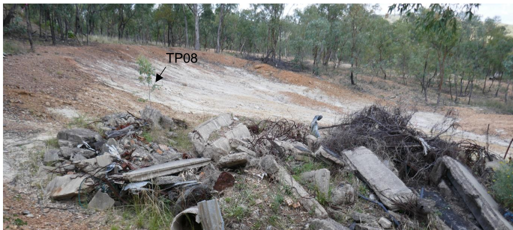
Image 5 Shallow excavation in sandstone at TP08
