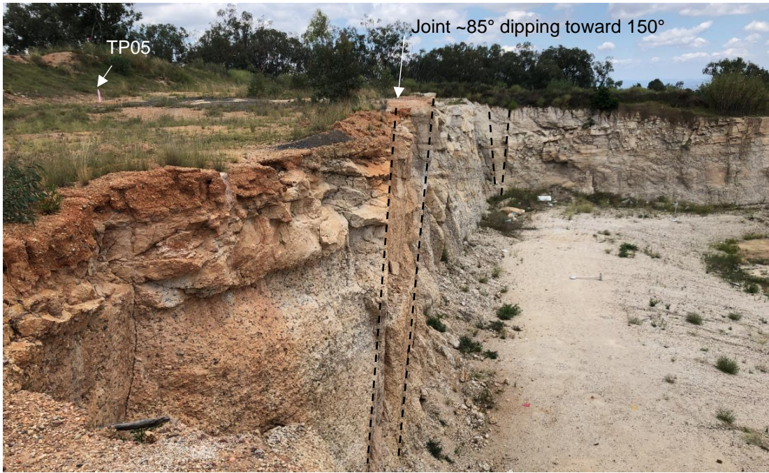
Image 9 Former quarry jointing
