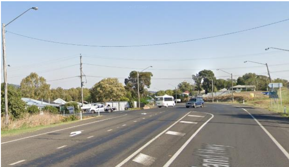
Figure 2.2 New England Highway looking north to Merriwa Road
